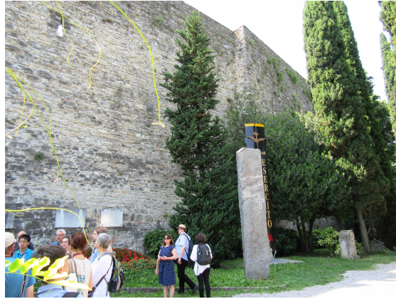
Bergamo: wall around the upper town
